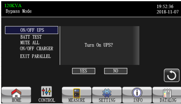
TURN ON UPS
